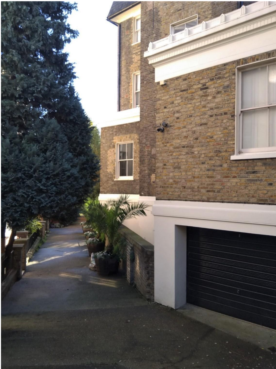
Side elevation of 26 Randolph Crescent as viewed from passageway
